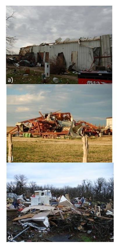
**Fig 3.** Photographs of damage caused by tornadoes on 29 December 2006. (a) Significant damage to a retirement home for veterans located outside of Groesbeck in Limestone County; (b) Damage to a metal framed barn east of Clifton in Bosque County; c) Remains of a mobile home destroyed by a tornado northeast of Rio Vista in Johnson County (Photo courtesy Gerald Mohr, Johnson County Emergency Management Coordinator).
