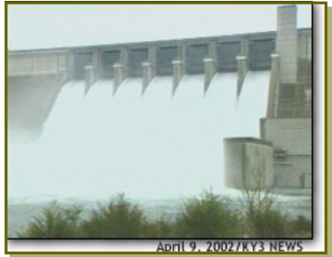
Spill way release gates open to ease lake level after heavy rains.
