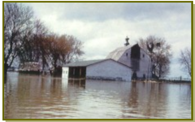
Flooding after heavy rains.
