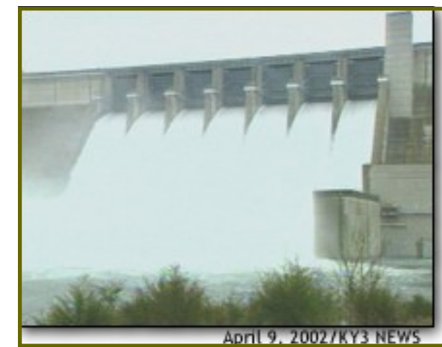
Spillway release of water after heavy rains
