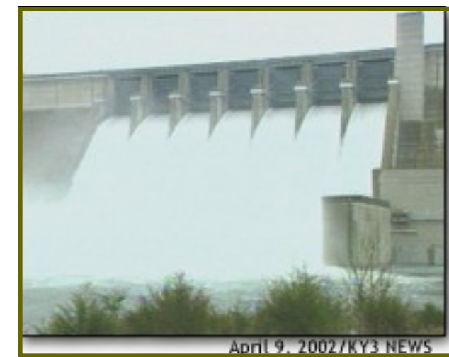
Spillway gates open to relieve lake level after heavy rain.
