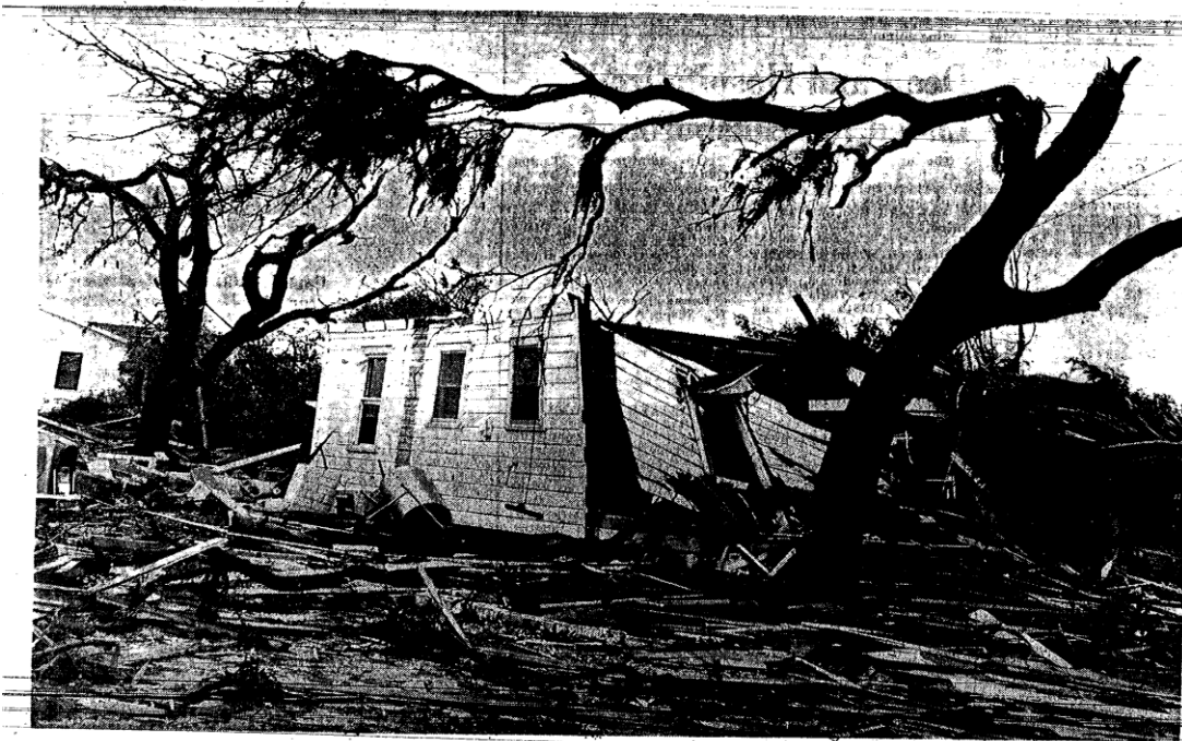
Walls collapsed on this house during the tornadoes fury Tampa Tribune
