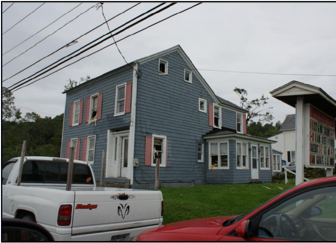
Figure 1: This home along Riverview Rd. in Cranesville had windows blown out, shutters damaged, blinds mangled and in disarray, and some roof damage, from the EF1 tornado. (NWS at Albany Photograph).
