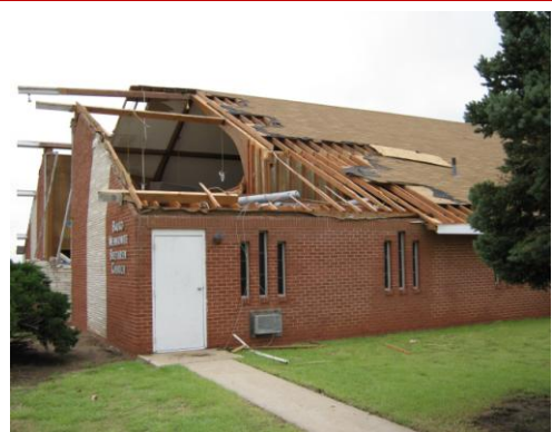
Church in Bryans Corners damaged on June 13 th .
