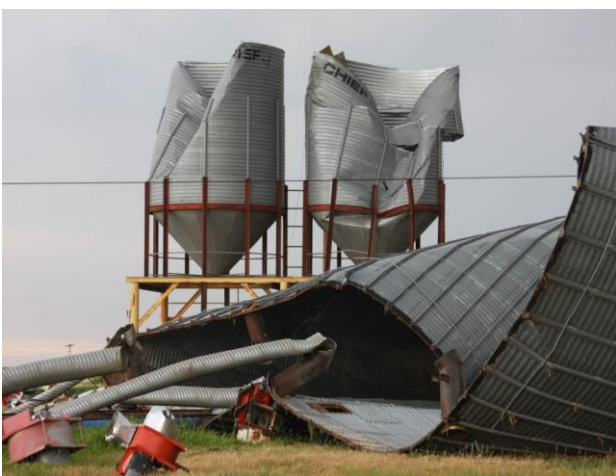
Grain bins in Bryans Corners damaged on June 13 th .
