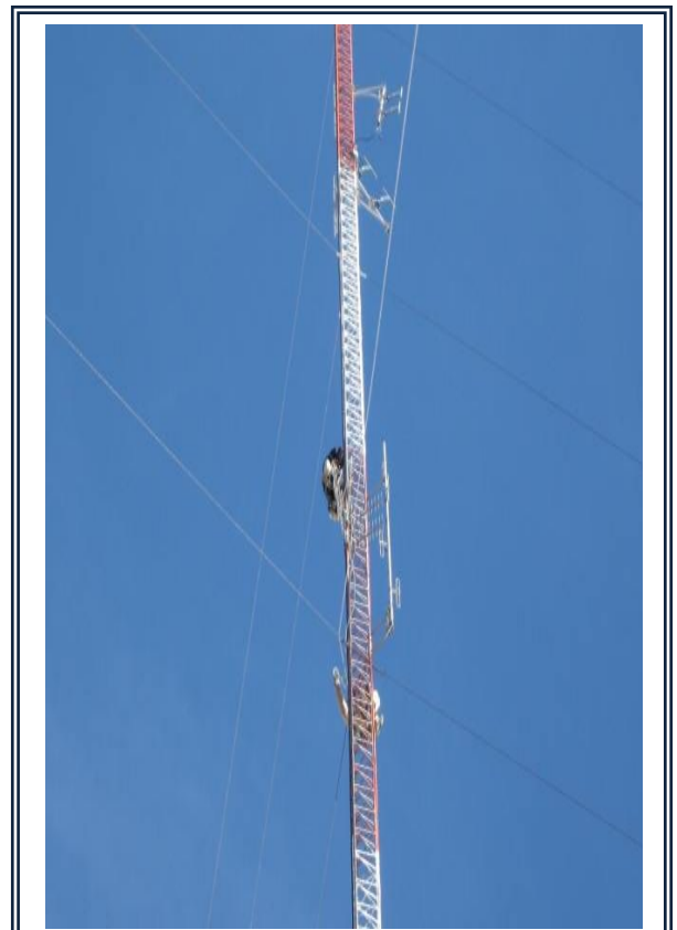
TRICO Tower employee working on the Perryton Transmitter
