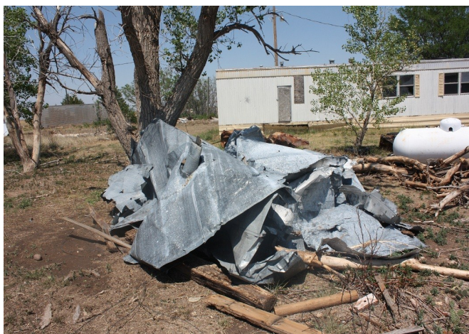
An EF-1 tornado blew the roof off of a manufactured home near Tyrone, OK on June 11.
