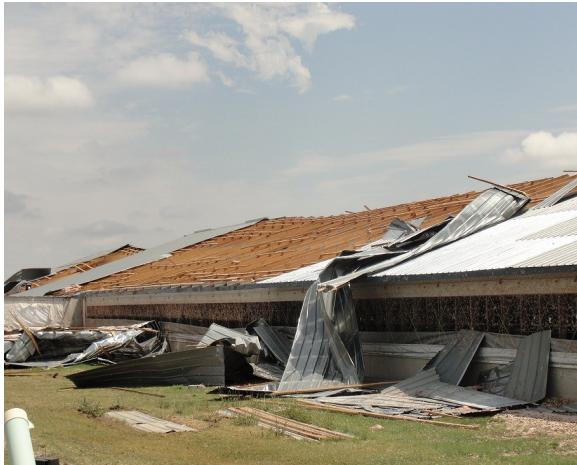
Straight line winds up to 120 mph caused significant damage to a hog farm on August 9, in Beaver County, OK.
