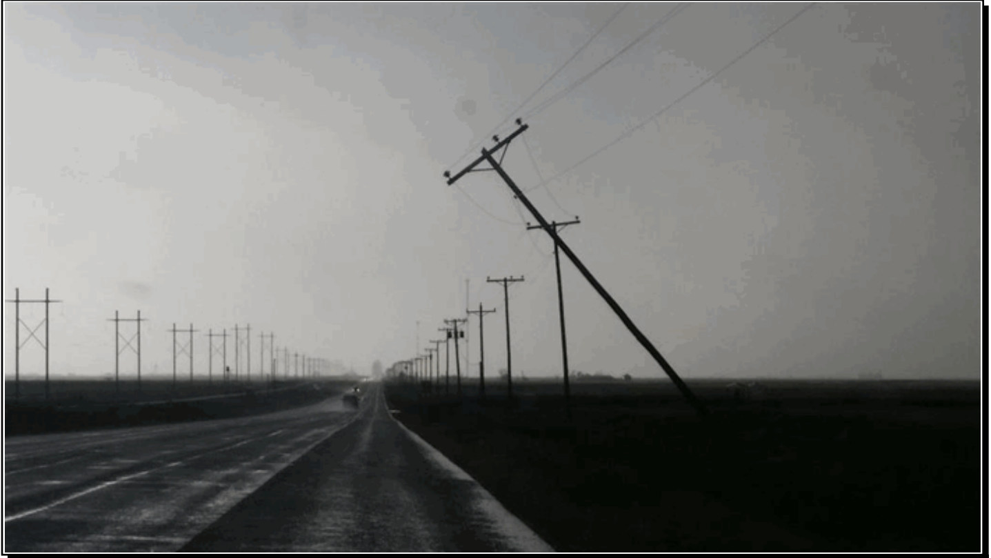
Power pole damaged by strong thunderstorm wind gusts just southeast of Hartley.
