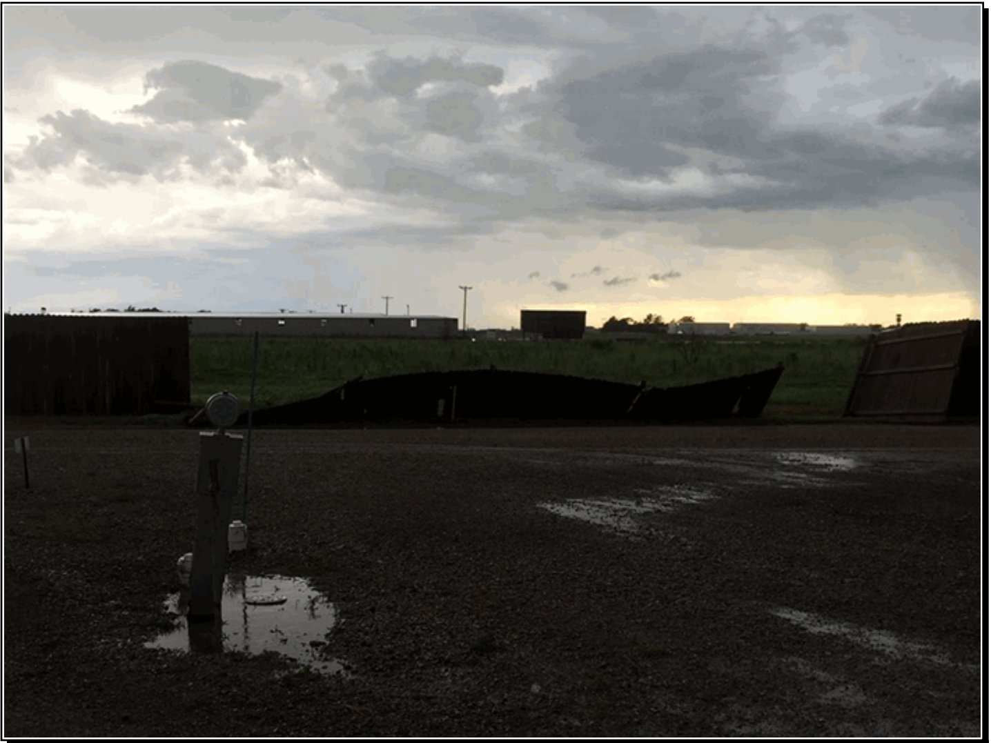
Damage to a wooden fence in Bushland from thunderstorm winds as high as 80 mph.
