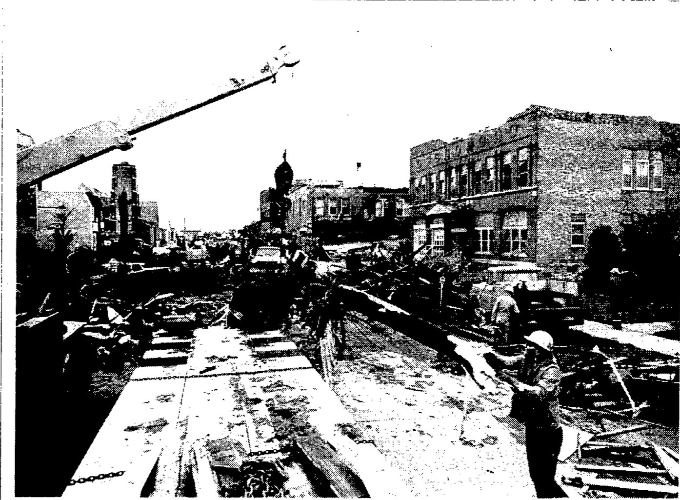
Stripped of its trees, First avenue NE at Oelwein emerged from a layer of rubble as workmen made "good progress" in cleaning storm debris from the city. Tornado funnels cut a large swath through the city shortly before 5 p.m. Wednesday, causing millions of dollars in damage and killing at least two persons. However, by Friday, most of the rubble was reported cleared away and the long, hard work of rebuilding was well under way. Oelwein's badly damaged city hall is shown at right.
