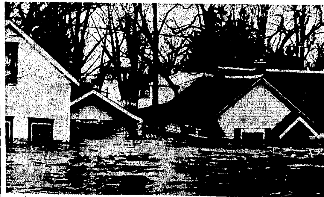
CROW RIVER RAMPAGE . . . The Crow River, cresting Wednesday at Delano, 25 miles west of Minneapolis, filled up the first floors of these houses along a residential section
