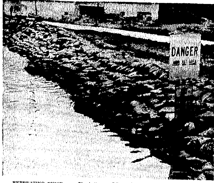
RETREATING RIVER . . . The bottom two rows of sandbags, wringing wet, were covered with water Wednesday morning. This picture was made where the Crooked Slough Dike and Prairie Island road connects, considered one of the danger spots in the dike system. (Daily News photo)
