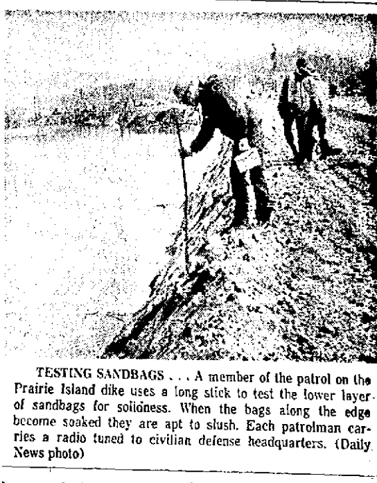
TESTING SANDBAGS . . . A member of the patrol on the Prairie Island dike uses a long stick to test the lower layer of sandbags for softness. When the bags along the edge become soaked they are apt to slush. Each patrolman carries a radio tuned to civilian defense headquarters. (Daily News photo)
