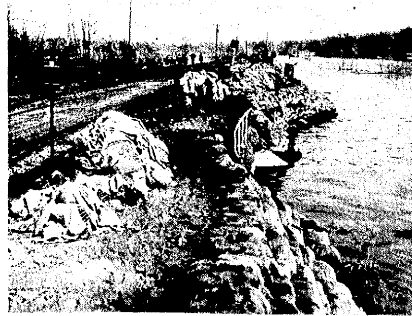
PRAIRIE ISLAND BRIDGE . . . On the downriver side the river is up to the top of the water entrance to Prairie Island gate bridge. The gates are closed now; earlier they were open to avoid too large a "head." The difference in level above and below the bridge can be seen by comparing the water heights in the picture. The big stack of filled sandbags is where the break came in 1952. Normally at this time of year this bridge is popular for carp fishing. (Daily News photo)
