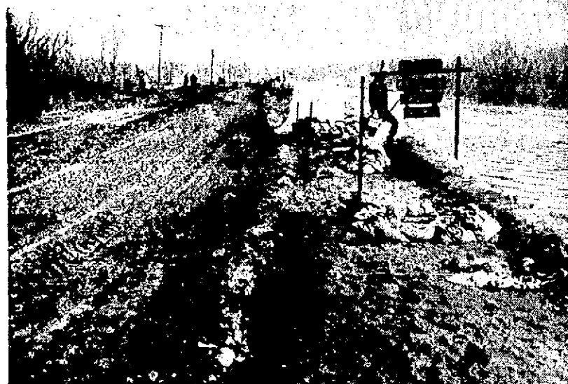
THREE LANE ROAD . . . The Prairie Island dike road has been raised five feet and widened to a three-lane highway. Big trucks moving over it have packed the surface to the hardness of city streets. Sandbagging crews and intensive patrol is being maintained. (Daily News photo)
