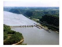
The US Army Corps of Engineers maintains a Lock and Dam (#9) at Lynxville, WI (below left) that is used to manage navigational water levels, not for flood control.
