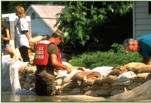
▲ Photo: Federal Emergency Management Agency
