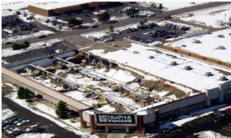
Figure 11. Collapsed roof of the large Bed, Bath, and Beyond store on south College Avenue in Fort Collins, CO. The roof on this structure was replaced and the store reopened several months later. Photo courtesy of Ron Phillips, City of Fort Collins.
