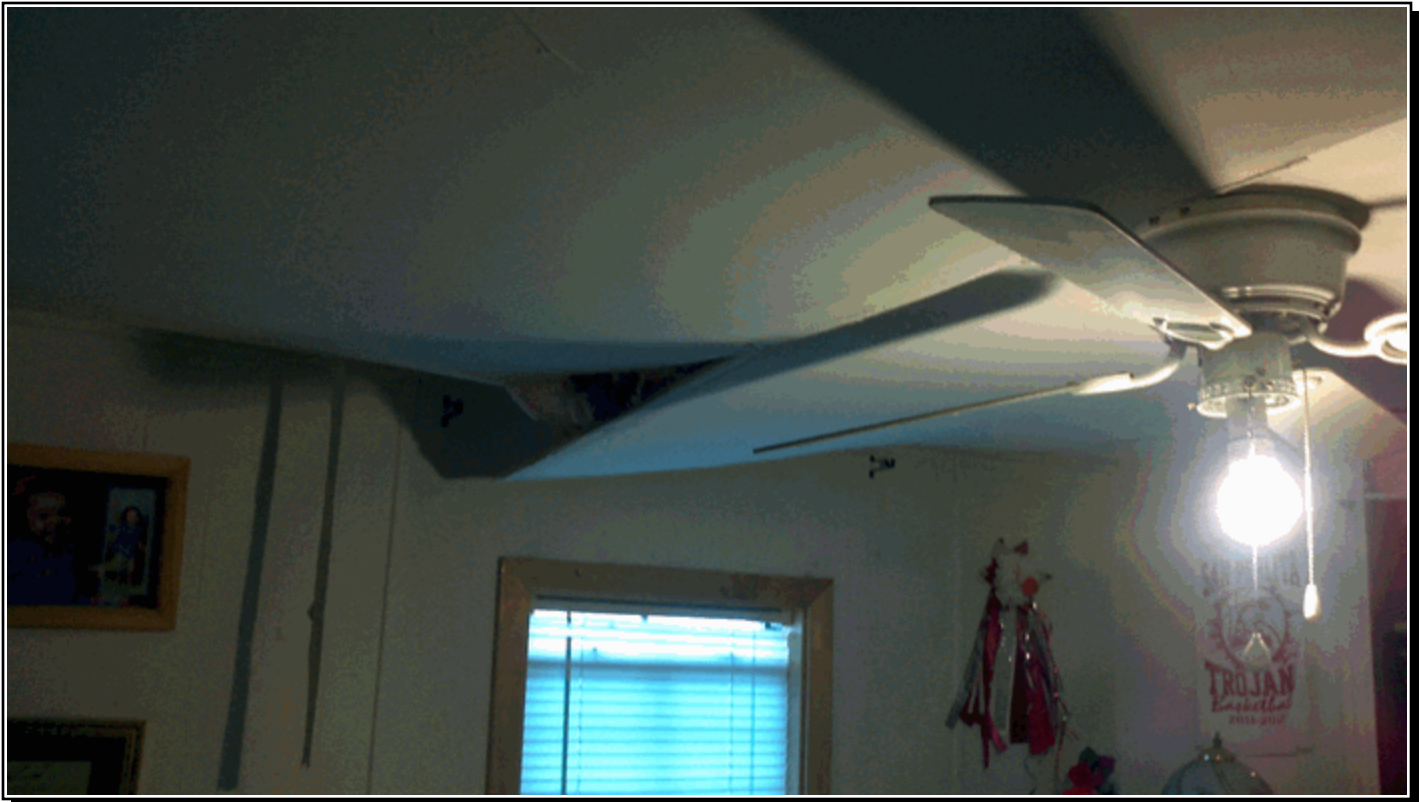
Roof damage to mobile home in San Perlita.
