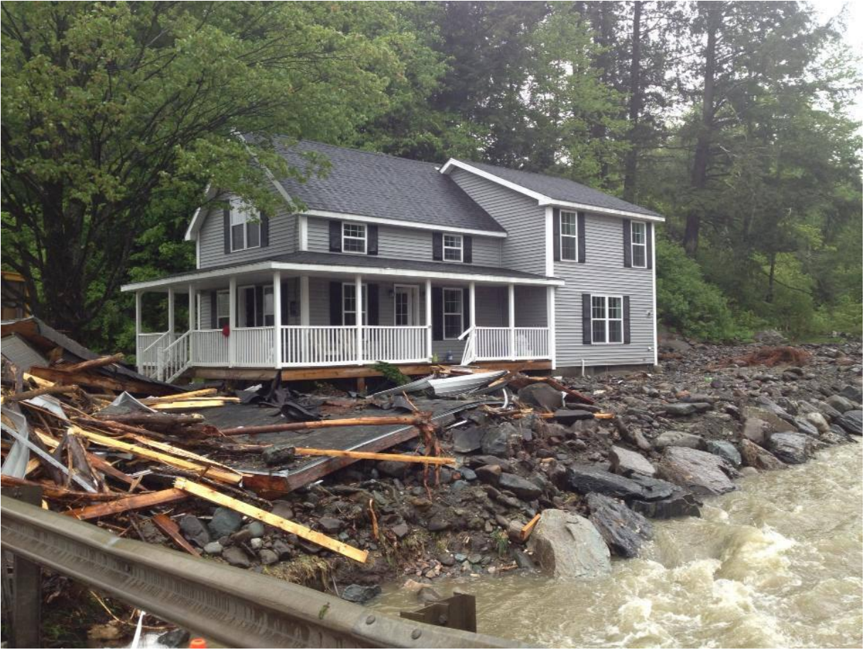
Figure 11: The intersection of Route 15 and Cilley Hill Road and associated damage from flash flooding.
