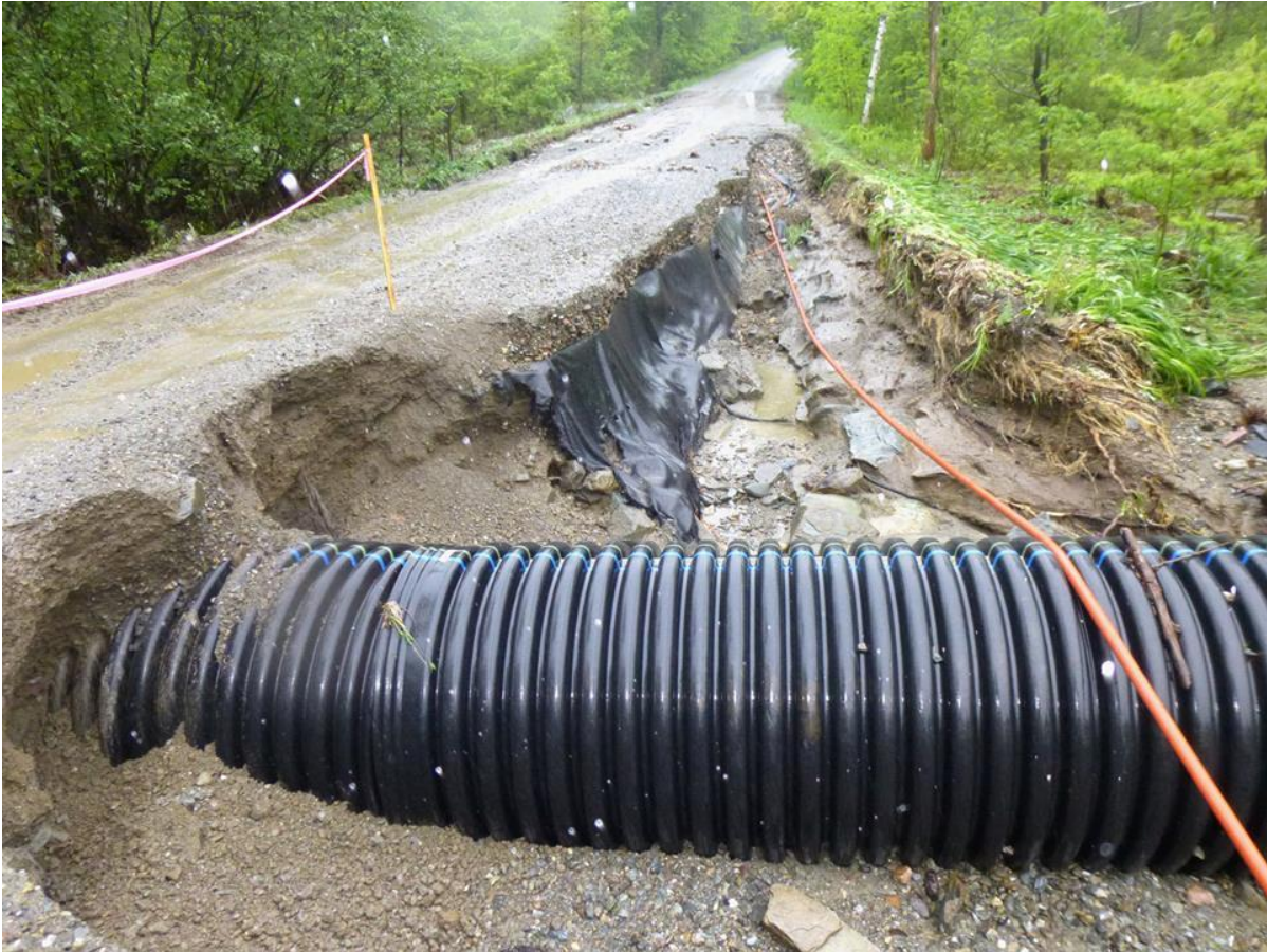
Figure 10: Flash flood damage on 23 May 2013.
