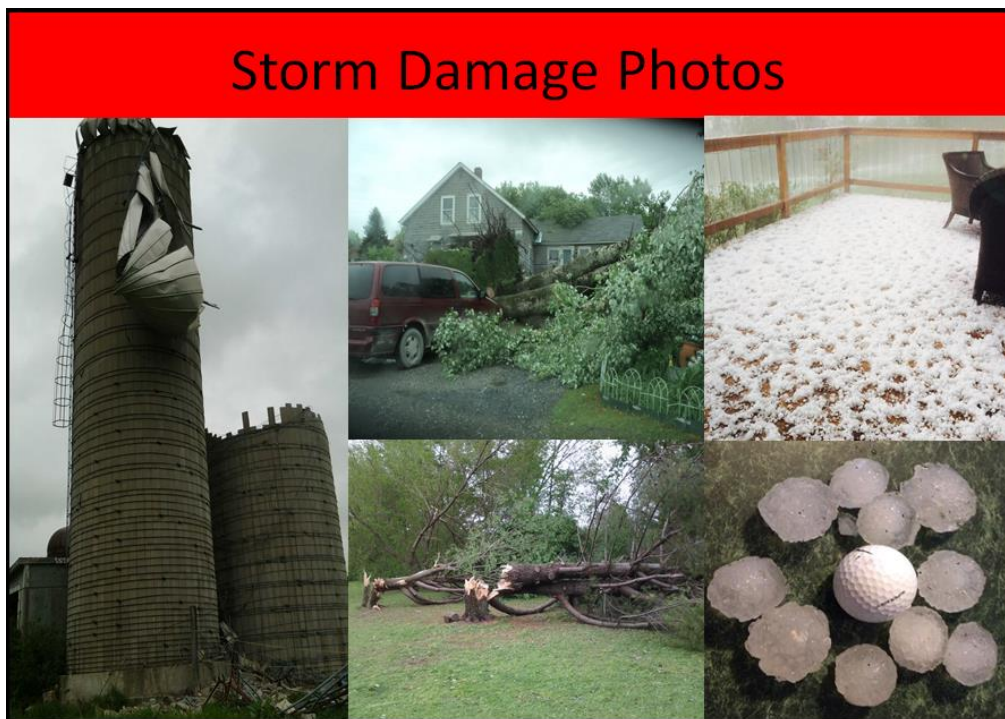
Figure 27: Storm damage photos from 27 May 2014.
