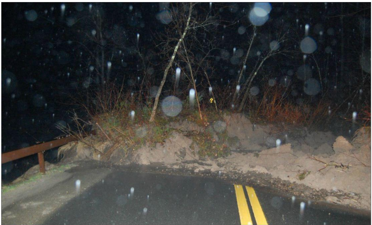
Figure 20. Debris slide, Stickney Bridge Road Jay, NY.
