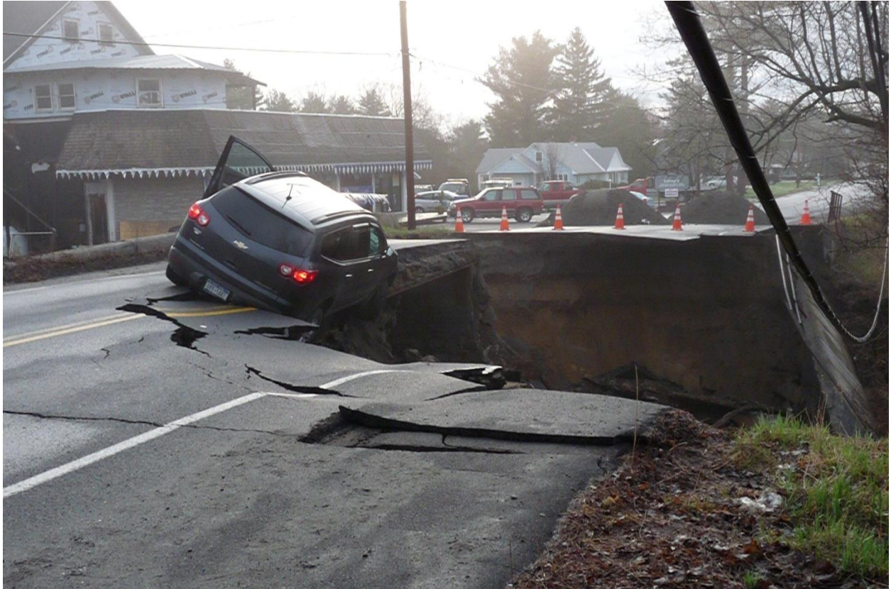
Figure 19. Broad Street bridge collapse, Moriah, NY.
