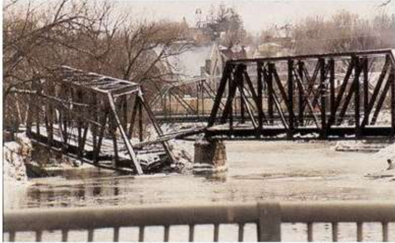
The pressure of the ice and water causes the Washington County Railroad bridge to snap.
