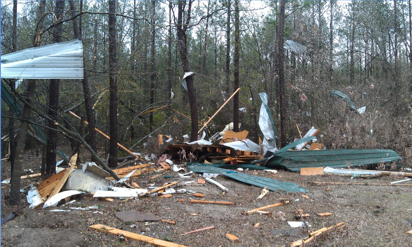
Damage associated with the tornado near Wagener
