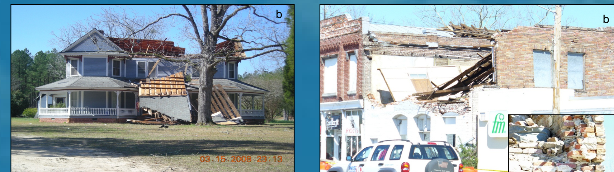
Figure 9: (a) GR2 Analyst radar imagery at 2108 UTC depicting the tornadoic supercell in Edgefield county, SC. 0.5 degree base reflectivity and cross section illustrate the classic hook, inflow notch, BWER, and elevated core. (b) EF3 damage to the top level of a two-story downtown Branchville, SC, building that was destroyed due to the tornado, note the inset picture of the triple-layer brick walls.
