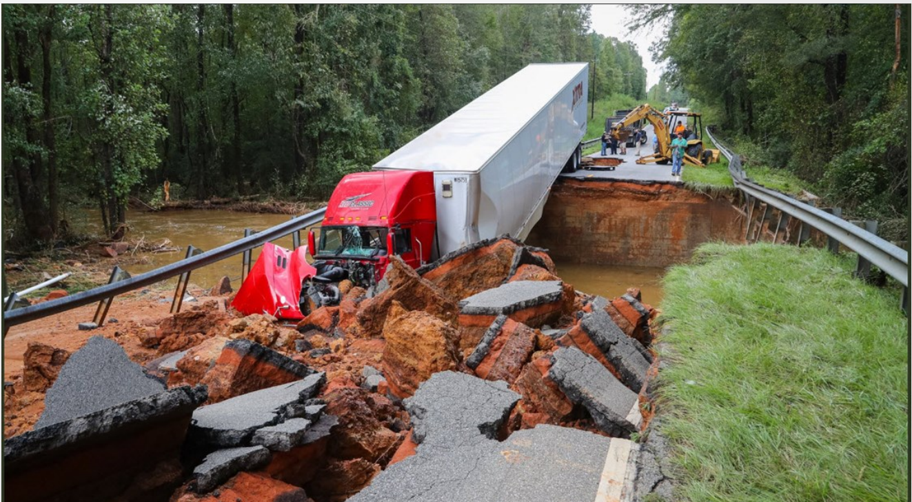
Hwy 145 in Chesterfield County SC washed out. (Photo courtesy Chesterfield Co. Sheriff)
