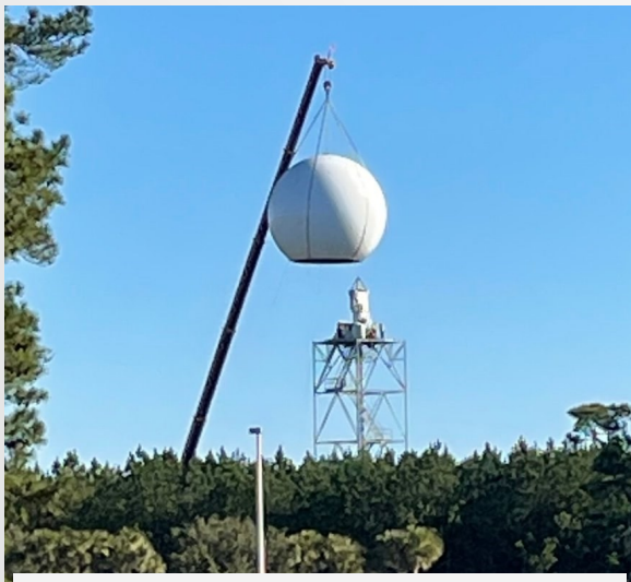
The crane lifts the dome protecting the radar to replace the pedestal.
