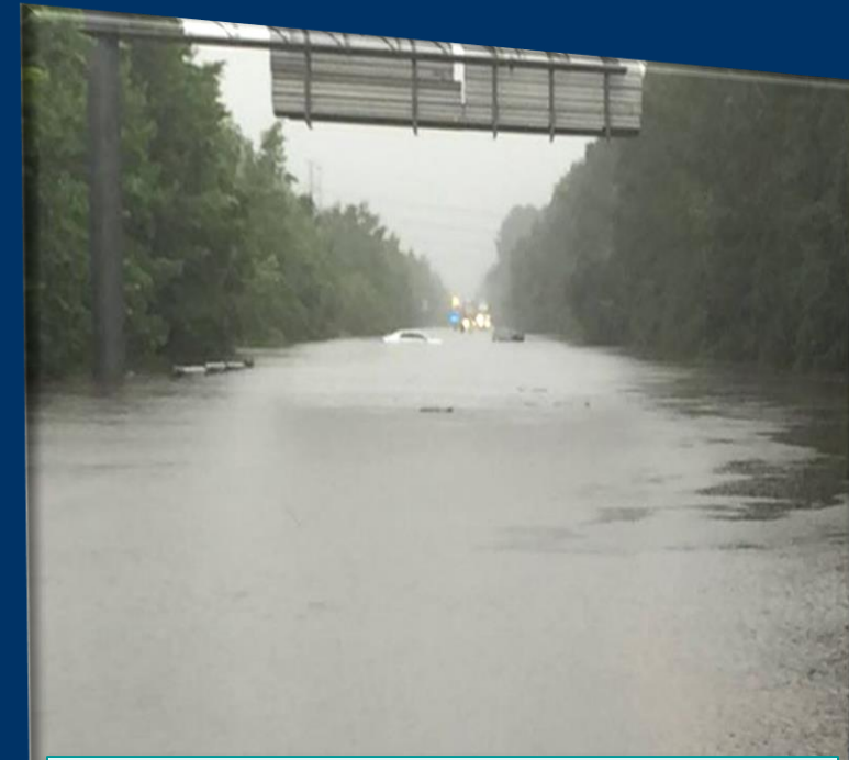
Flooding on Interstate 95 from Tropical Storm Bonnie (2016)
