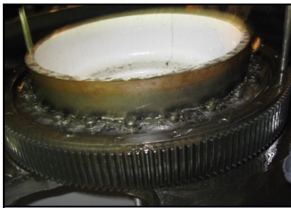
Damaged Bull Gear
