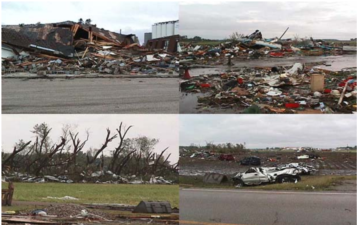
Figure 3. Photographs taken by a National Weather Service storm survey team, showing tornado damage up to EF4 intensity in Northwood, North Dakota.
