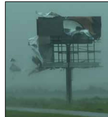
Above: Wind damage to a billboard from Hurricane Lili in October 2002.
