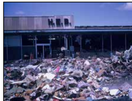
Wind damage from Hurricane Celia
