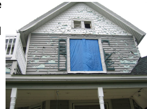
Hail damage in Eldora, IA.
