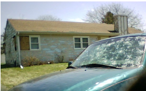
Hail damage in Eldora, IA.
