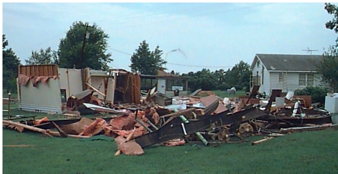
A mobile home was rolled off its foundation due to straight-line winds associated with a severe thunderstorm in Alabama.
