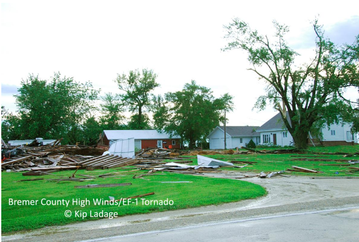
Destroyed barn at Point 2. Picture is courtesy of Kip Ladage.
