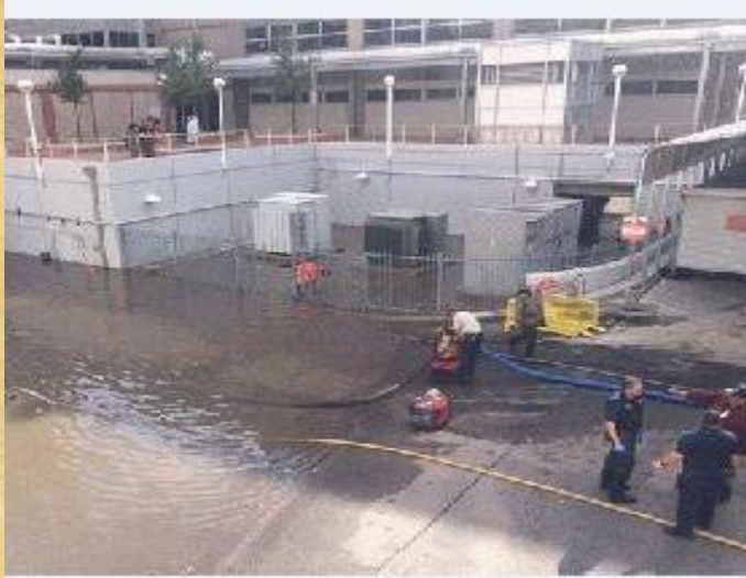
Univ. Med. Center Flooded
