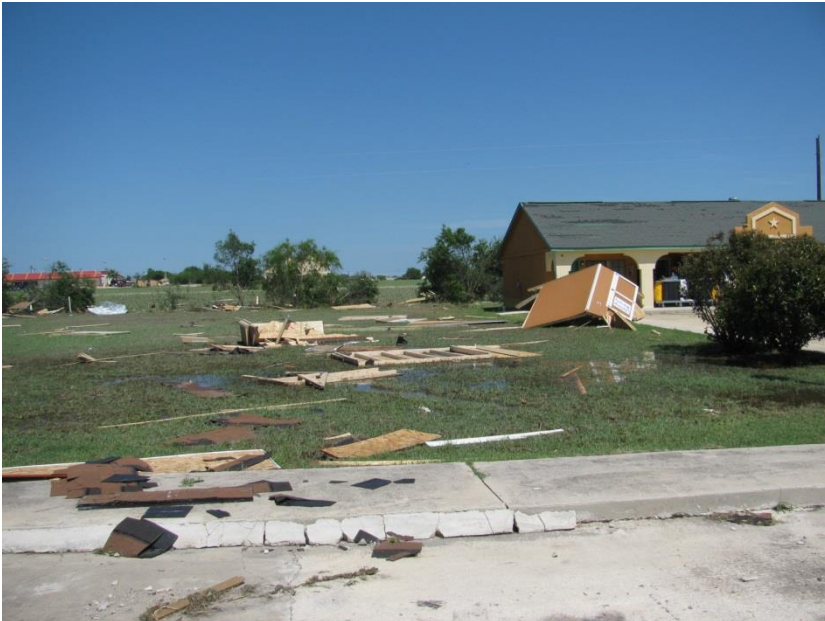
Pieces of at least 2 wooden sheds in Hondo, TX (Photo Credit: NWS)
