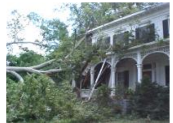
A small sample of the damage done by Hurricane Frances. This damage occurred in Morgan County on Sept. 7th.
