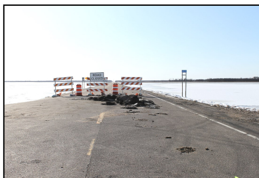
Figure 24 Closed Road west of Stephen, MN
