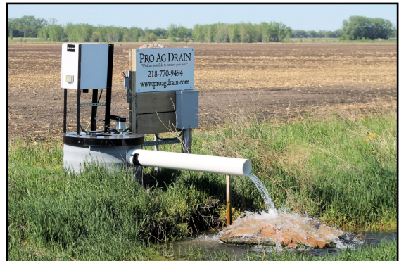
Figure 23 May 27, 2020 Drain Tile Pump Near Arvilla, ND
