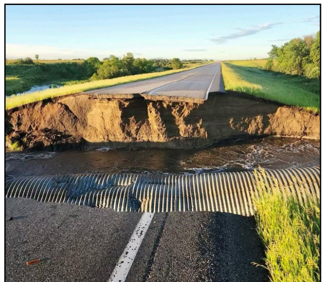
Figure 21 Washed out road 9N of US Highway 2 on ND32
