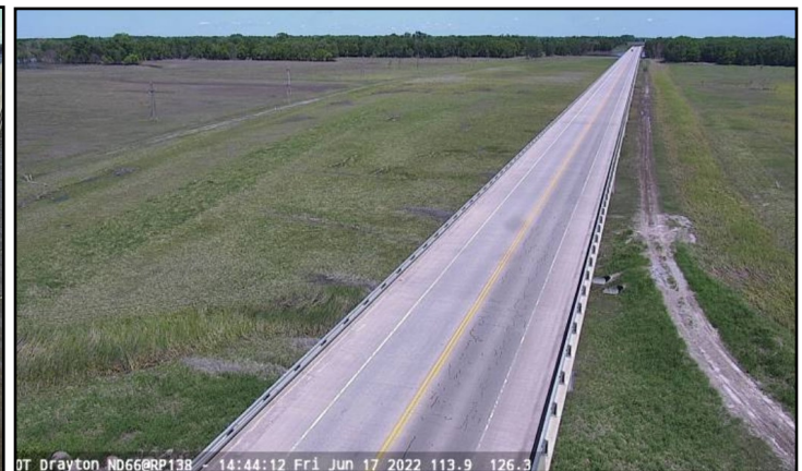
Figure 25 Drayton ND Red River Bridge June 17th
