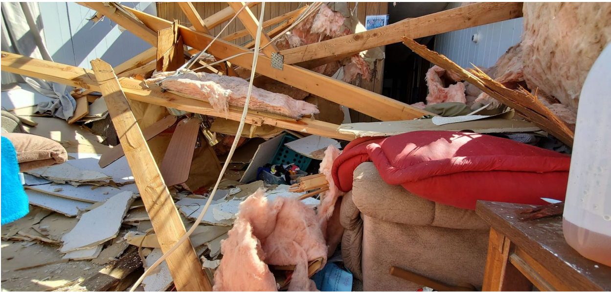
The center of this photo is in the living room and where the person was pinned after half the roof was blown off and some of the trusses collapsed into the home.
