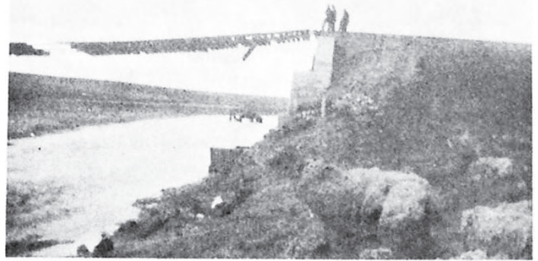
1935 Flood waters under Vona bridge (railroad).
