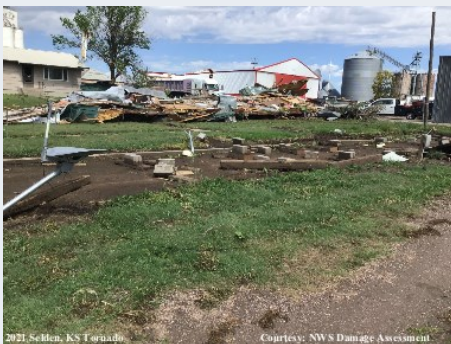
Damage to a mobile home from the Selden, KS tornado on May 24th, 2021
