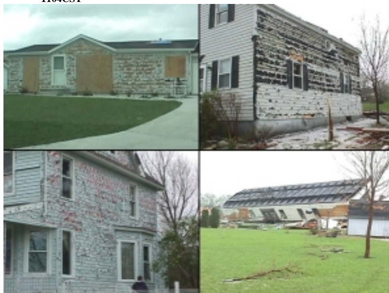
Hurricane-force winds, combined with golfball and baseball size hail, produced extreme damage to homes and businesses in Calumet and Manitowoc counties.
