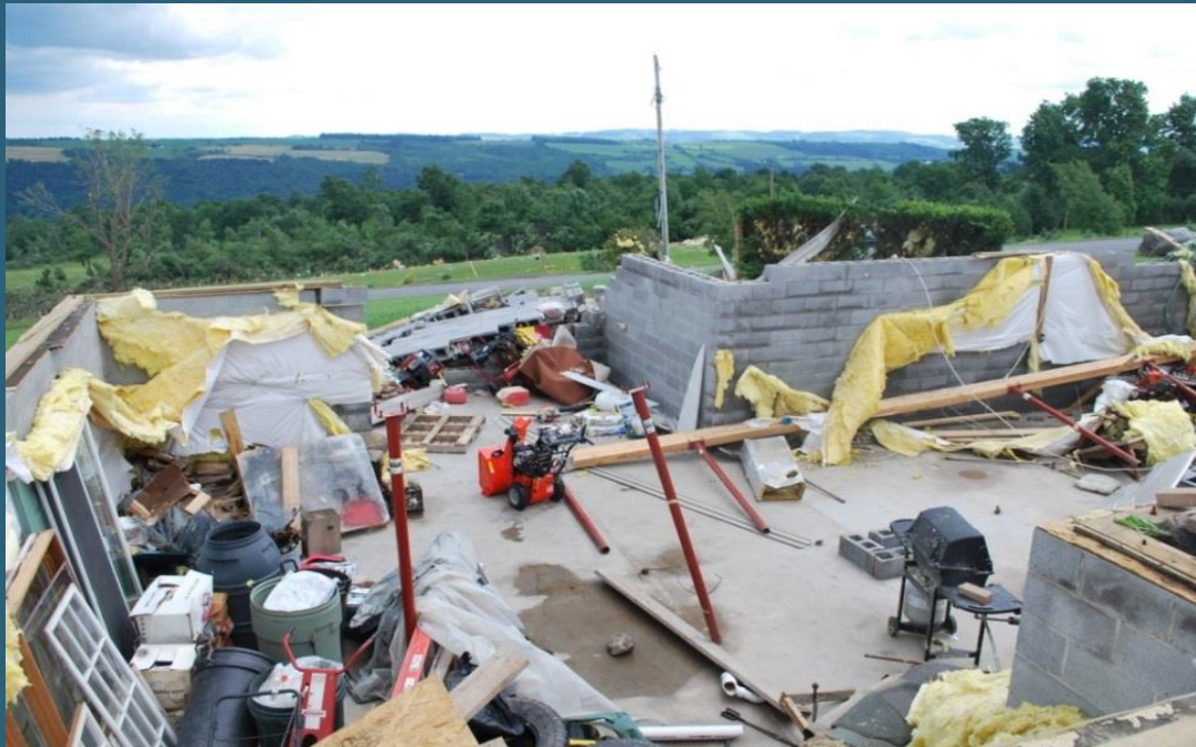
Damage near Smithfield, NY
