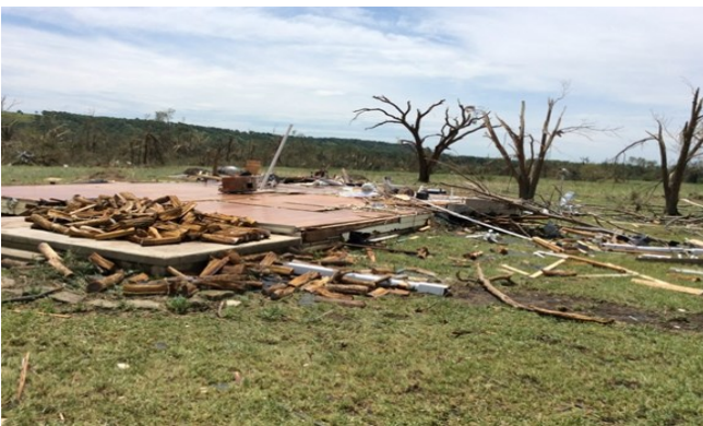
The remains of a residence that sustained a direct hit. Note the significant tree damage as well. Photo courtesy of NWS Wichita damage survey.
