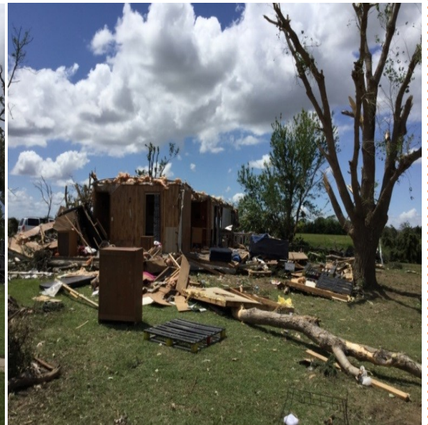
EF3 damage 2 miles west/northwest of the Great Bend Airport
