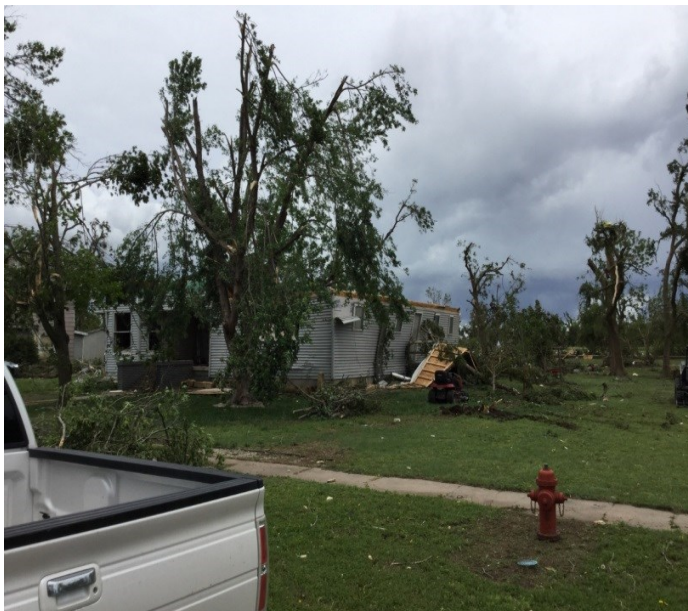
EF2 damage on west side of Pawnee Rock
