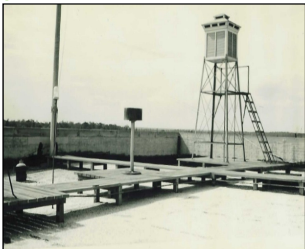
Official weather observing equipment on top of the Customs House Building along Water Street in Downtown Wilmington, 1934.
