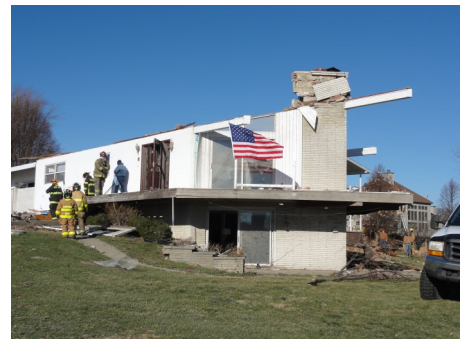
This house was damaged by an EF-3 tornado which moved across the Lake Petersburg area of Menard County on New Year's Eve 2010.
