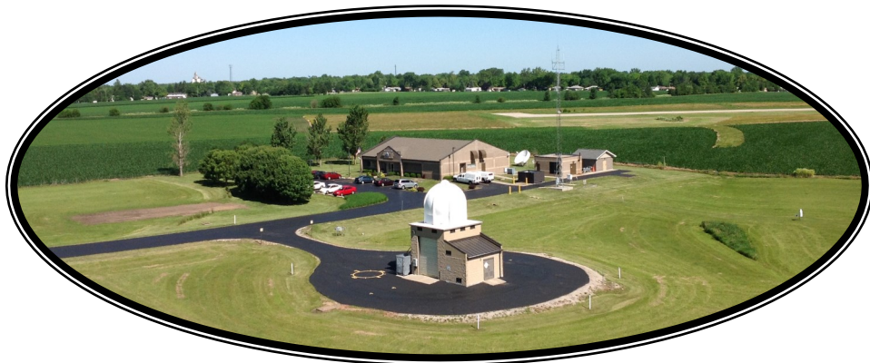
The Lincoln NWS office as seen from the radar tower, June 2014.
