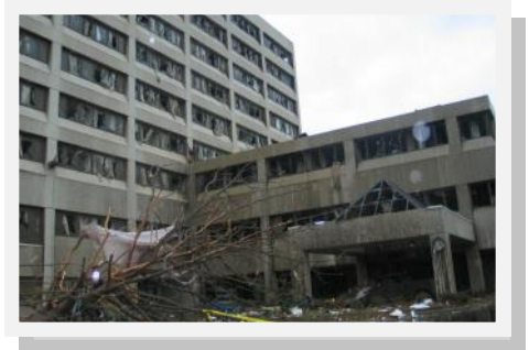
Damage to St. John's Regional Medical Center in Joplin, MO, on May 22, 2011. Photo by NWS Springfield, MO.
