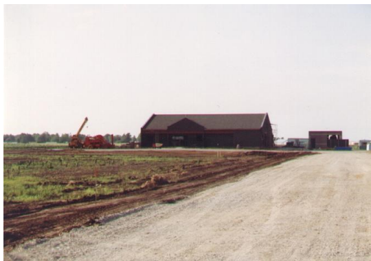
Construction of the new Weather Forecast Office in Lincoln during 1994.
