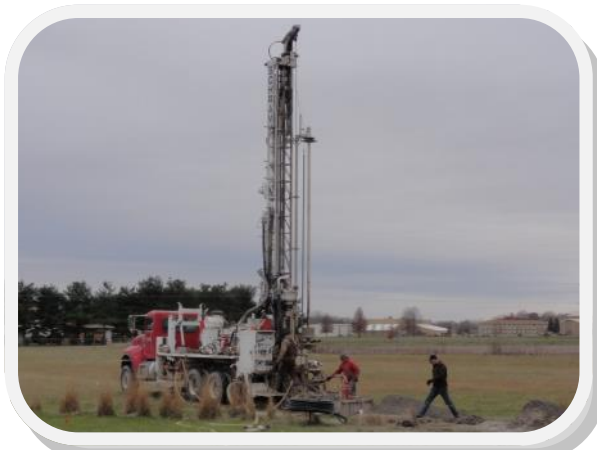
Workers drill holes in the land in front of the NWS office on November 25, as part of the installation of a geothermal heating system that is being installed.
