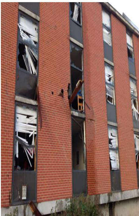
Outside walls of a home in Panola County, collapsed after being struck by an EF3 tornado. Interior walls remain standing (above). Two large wooden boards pierced brick walls of a building on the campus of William Cary University near Hattiesburg, MS. (left). Both of these photos reiterate why being in the interior portion of a home/building is important, and why wearing a helmet is a good idea!
