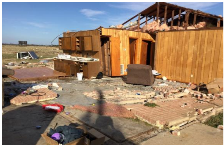
Outside walls of a home in Panola County, collapsed after being struck by an EF3 tornado. Interior walls remain standing (above). Two large wooden boards pierced brick walls of a building on the campus of William Cary University near Hattiesburg, MS. (left). Both of these photos reiterate why being in the interior portion of a home/building is important, and why wearing a helmet is a good idea!
