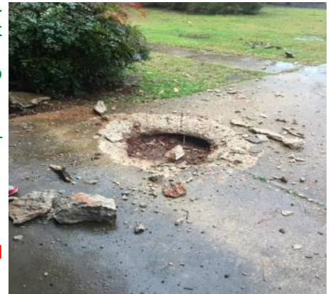
A lightning strike caused extensive damage to this driveway in Magee, MS. Photo by: Chris Curlee
